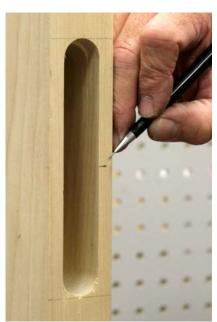
Make a mark at this point, this will be the center of the mortise pocket and the center of the mortise faceplate.
