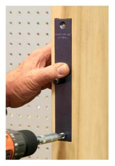
The second half of the template will attach to the faceplate area. Use a self centering drill to locate the screw holes required by the mortise lock. This will help with alignment and prevent binds when the lock is installed. Use the factory supplied screws to attach to the door.
