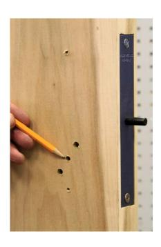
Once all holes and pilot holes have been drilled, enlarge per the mortise lock specifications. In this example the spindle hole is being enlarged from the 1/4" pilot hole to the required 1-1/8" size. Drill all other holes in the same manner.
