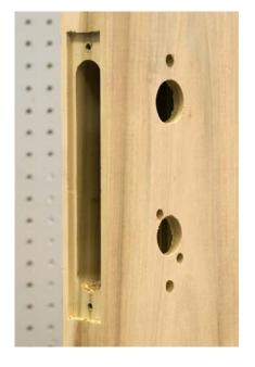
Completed installation, install mortise lock per factory instructions.
