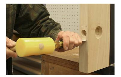
A chisel can be used to deepen the top and bottom of the outlined area. Once everything has been outlined, chisel out the latch mortise.
