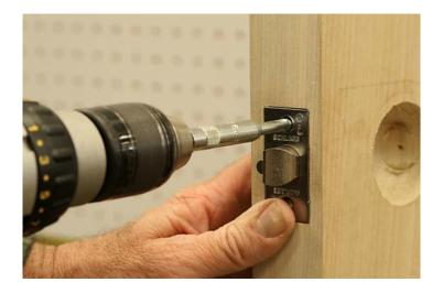
Use one of our centering drills to drill for the latch screw. This will assure a centered hole and will allow you to drive in the screw with out splitting the door. Do not attempt to drive in a screw without a pilot hole.
