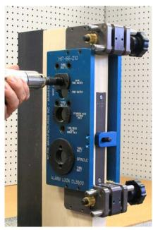
With a 3/4" hole saw, drill the wire run hole. This hole goes through the door and is drilled half way from both sides of the door.
