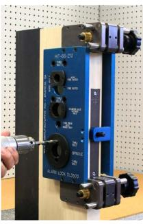
Start by drilling all of the required 3/8" diameter holes used for the thru bolts. We are drilling the lower holes above and below the mortise lock spindle hole. These holes go to the mortise pocket. Use a standard twist drill for wood or metal doors.
