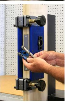
Start by drilling all of the required 5/8" diameter holes used for the thumb turn and escutcheon trim. A brad point bit can be used on a wood door, or a hole saw may be used on both wood or steel doors.
