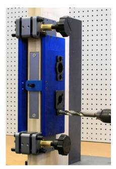
The top and bottom 5/8" diameter holes for the escutcheon trim are being drilled in this step. Be sure to drill only half way from both sides of the template. In the picture we are using a brad point bit, a quality hole saw may also be used on both wood and metal doors.
