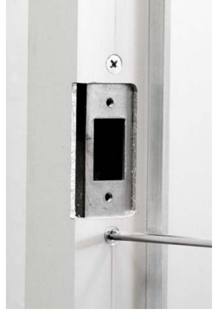
Finished installation showing strike and dust box.
