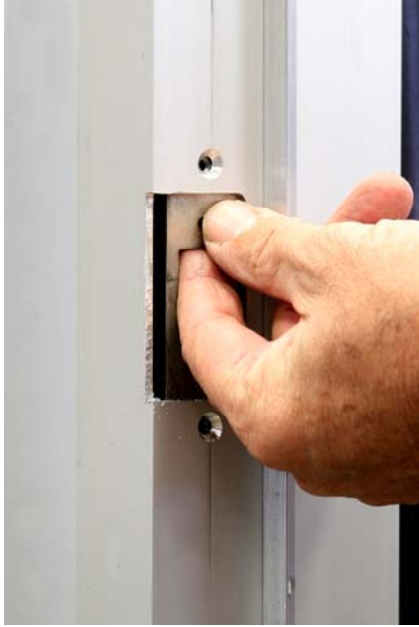
Factory mounting bracket being installed.
