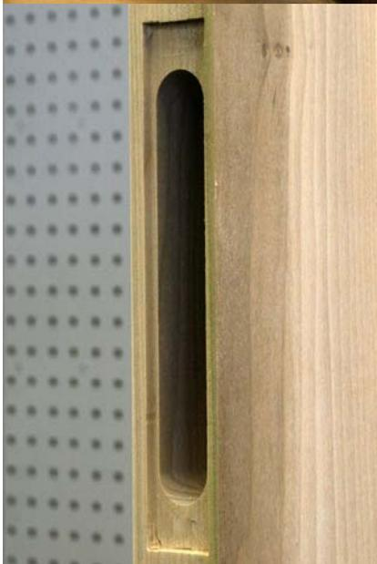
Shown is a standard mortise pocket, we will use this as a basis for the Onity install. If the holes for the mortise lock are not drilled, use the HIT-4509 alignment fixture and a center drill to drill the pilot holes. Do not try to “eyeball” the center and drill a hole or use an awl.
