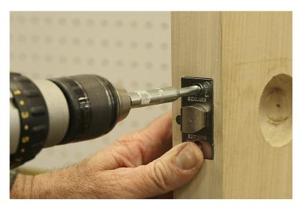
Use one of our centering drills to drill for the latch screw. This will assure a centered hole and will allow you to drive in the screw with out splitting the door. Do not attempt to drive in a screw without a pilot hole.
