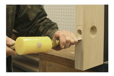
A chisel can be used to deepen the top and bottom of the outlined area. Once everything has been outlined, chisel out the latch mortise.
